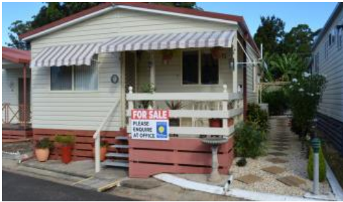
Unit 11, 210 Pacific Highwa, Coffs Harbour, NSW
