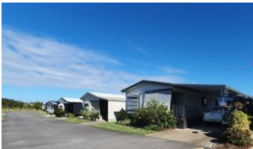
CT 40 69 Light Street, Casino, NSW
